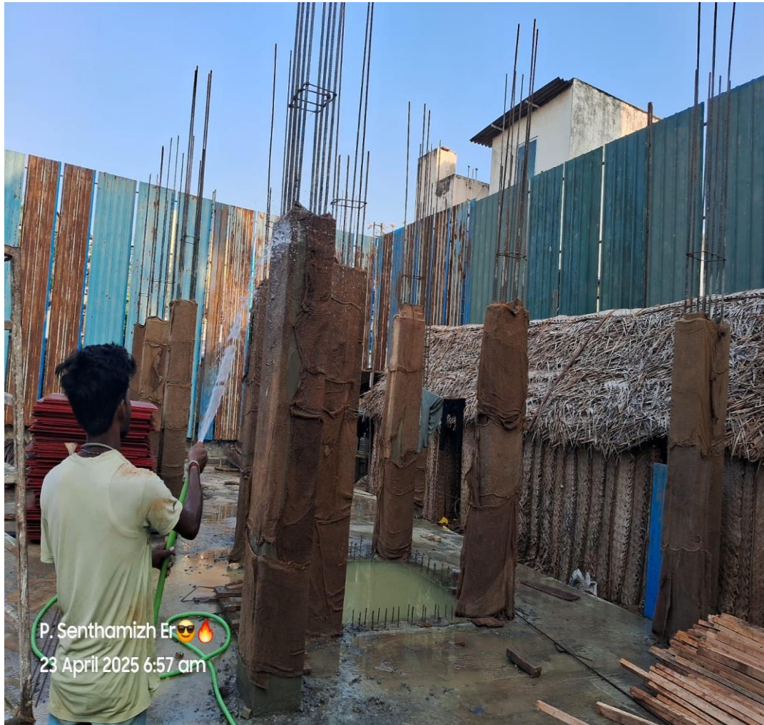
Stilt Floor Grade Slab RCC & Column RCC WIP
