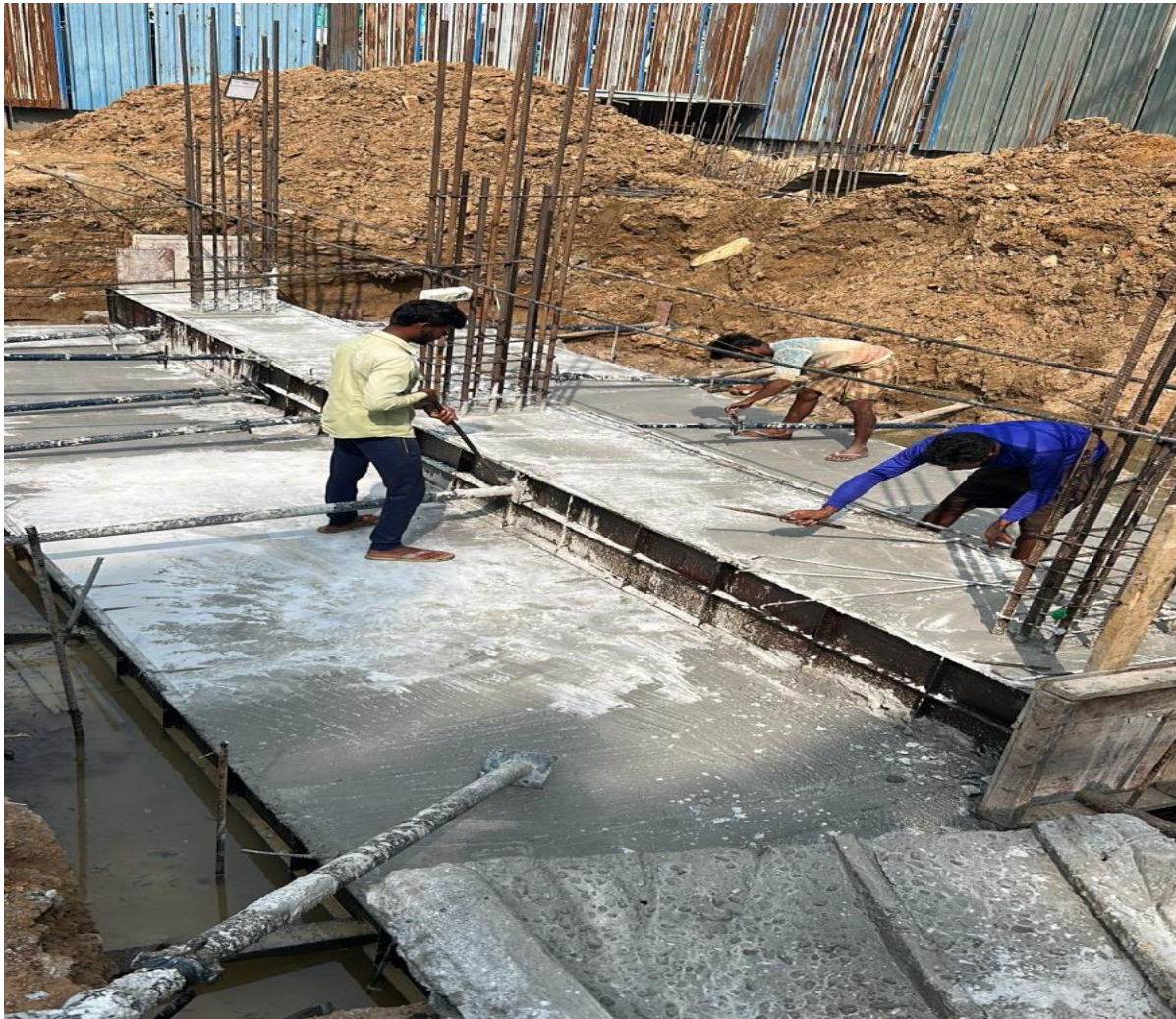
Footing Shuttering & RCC Works
