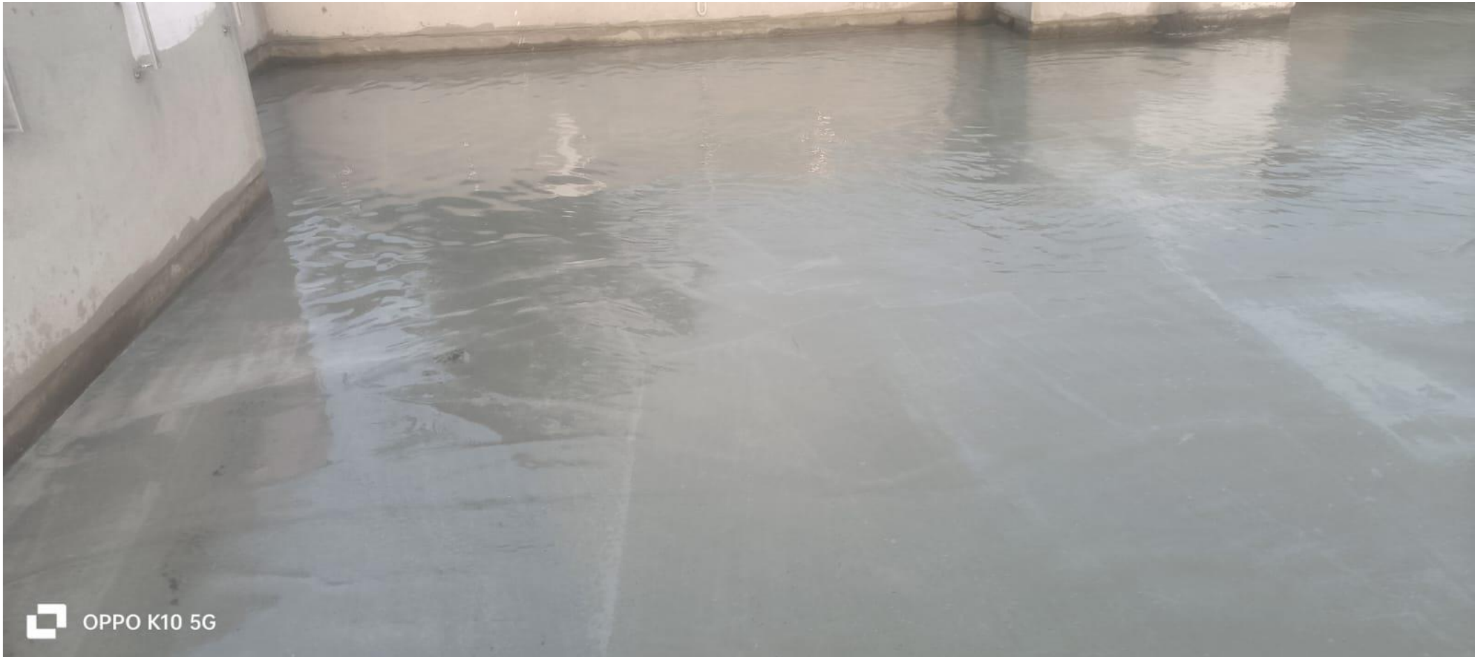
G+4 Residential Apartments – Nu – Tech Sri Krishna – Nearing Completion Stage – Terrace Floor Screed Concrete
